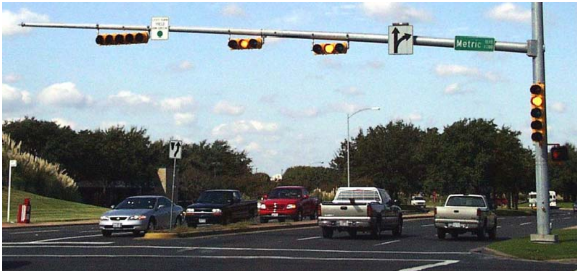
Figure 1-1: A Typical Mast Arm Signal Structure (Anderson, 2007)
